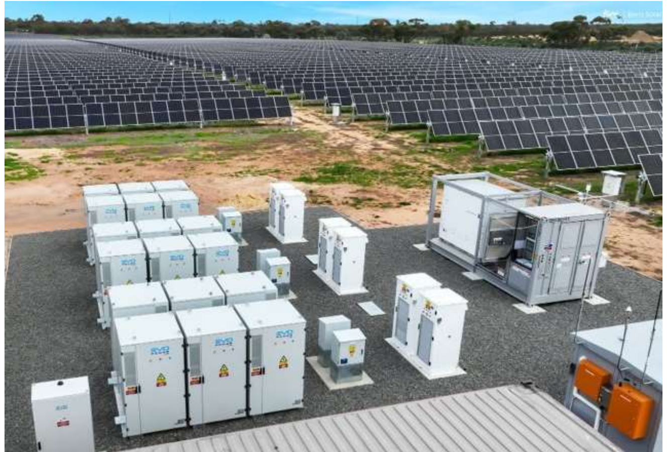
5.8 MW solar with 3 MW battery at Berri
