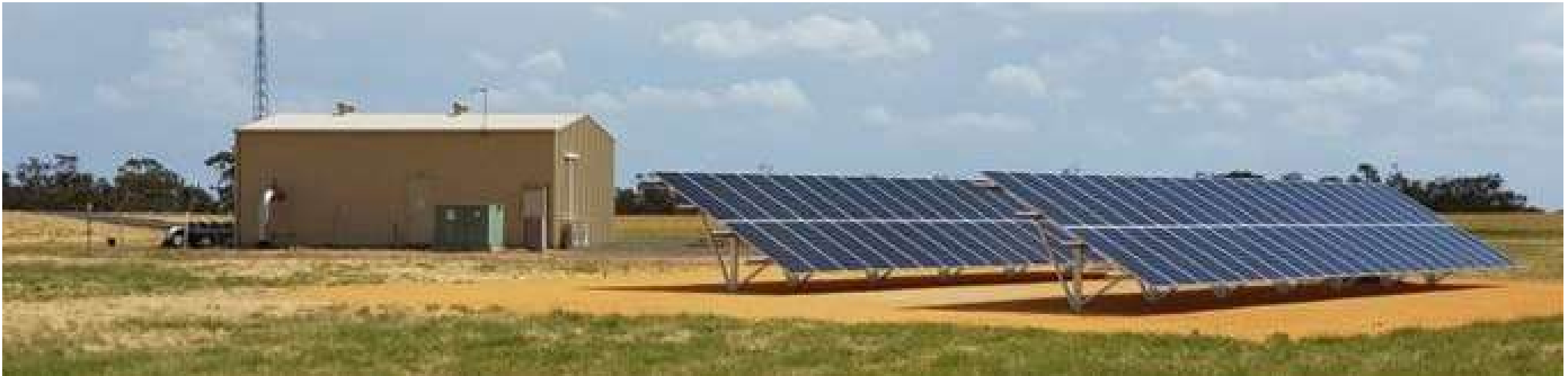
Solar installation at Dimboola pump station
