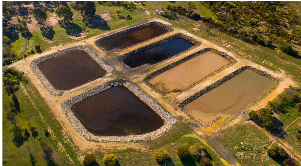
Lagoon-based wastewater treatment facility
